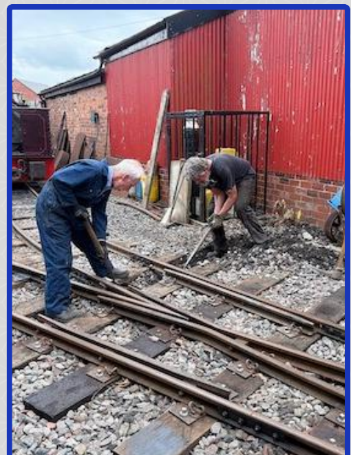
Arthur and Andy get busy laying a cableway for the planned solar panel installation.
