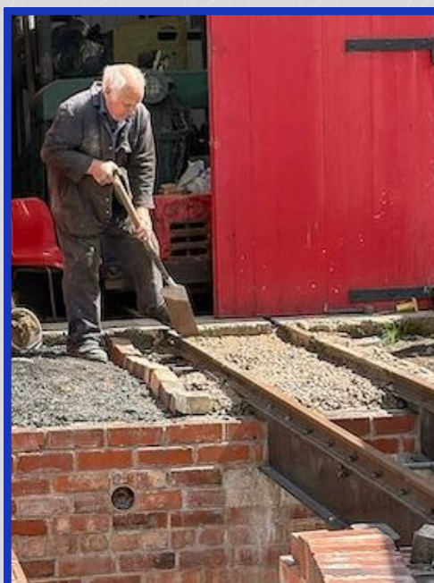
Paul beds in the rails for the new ash pit, now nearing completion.
