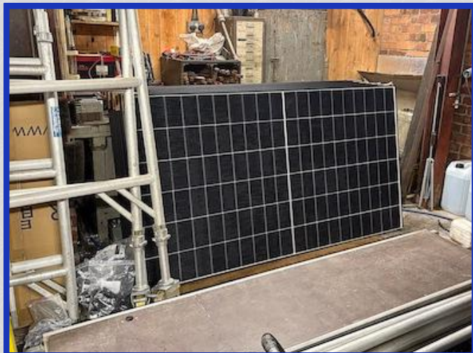
Thanks to a grant from the Lancashire Environmental Fund we have obtained solar panels for the new workshop roof.
