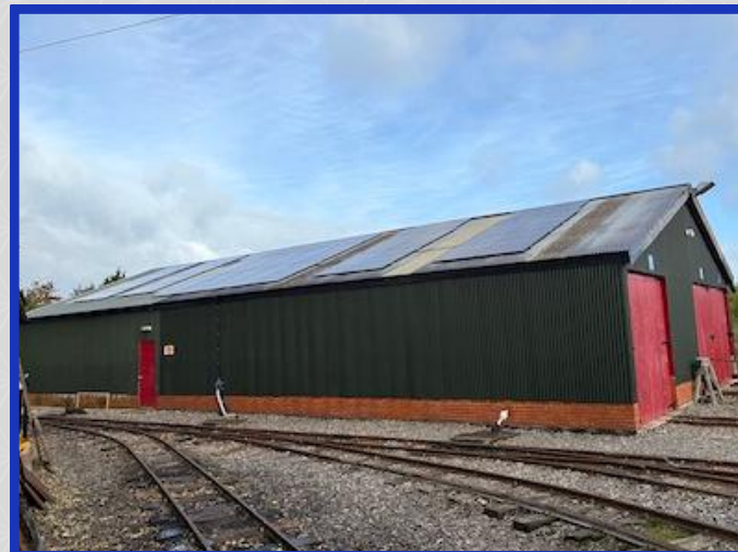
The panels installed and working, making a significant contribution to our energy supply.
