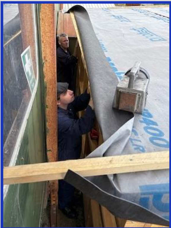
Mike and Arthur were specially chosen to fit in a tight corner, adding a waterproof membrane to the model railway shed.
