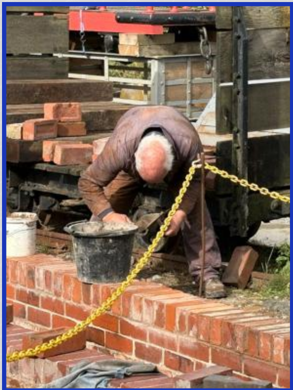
Paul demonstrates prowess with hawk and trowel, topping-off the walls for the new ash pit.
