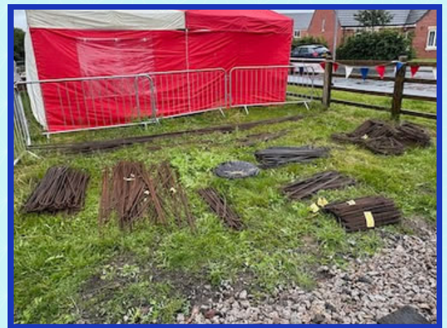
Delivered and sorted, ready for the construction crew.
