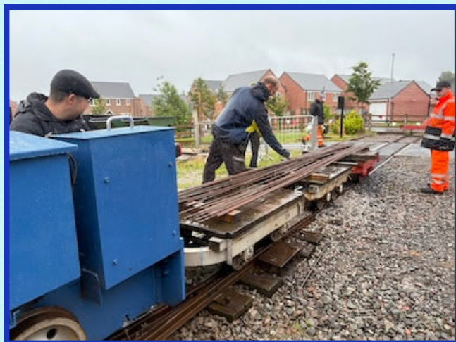
A ready-made transport system moves the reinforcing bars for Y Caban .
