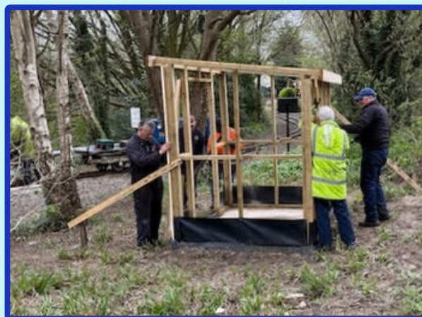
Good progress on the Squeal Shed, to house the equipment for watering dry rails on the curve near Delph.
