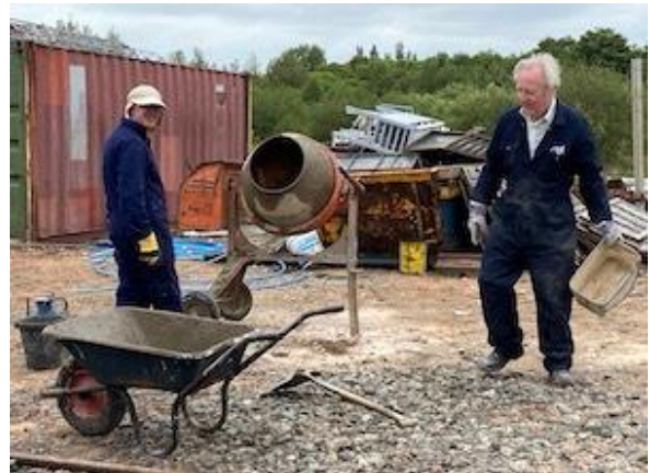
...while Andy (2) and Adrian mix the concrete, with some mechanical assistance.
