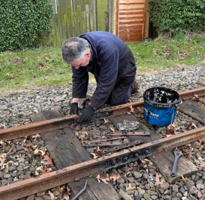
Another important job is lubricating the fishplates that join the rails together. Mike leads by example, ruining yet another pair of gloves in the process.
